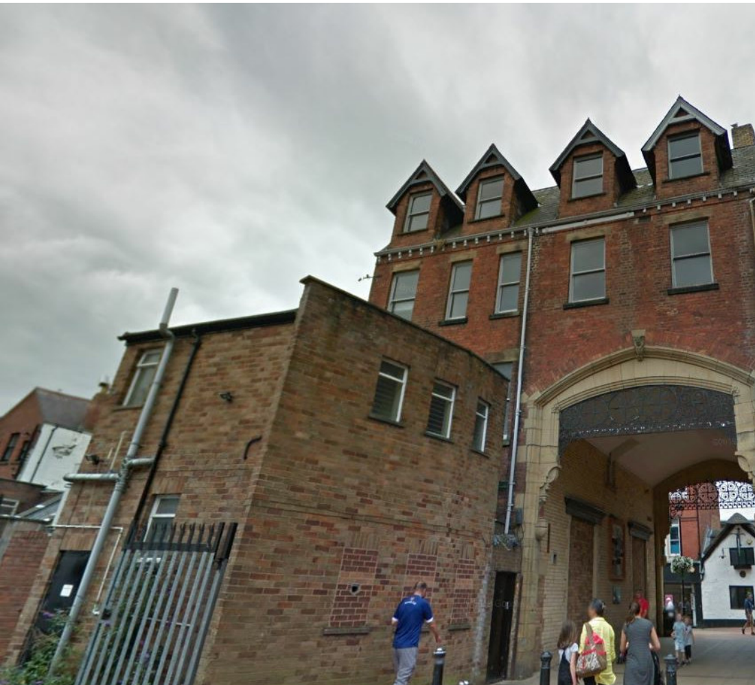
Rear Elevation from Argyle Street
