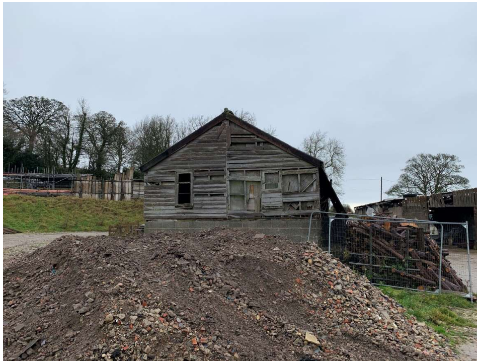
Photograph 1; rear gable showing surrounding farmyard
