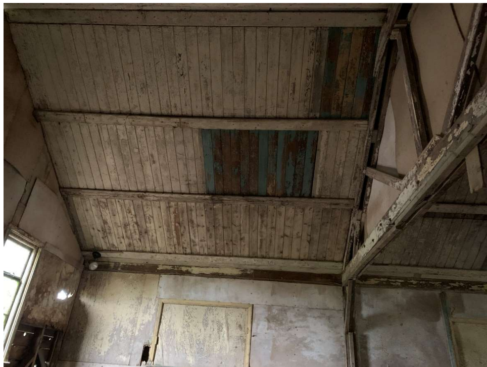
Photograph 6; timber sarking boards in good condition
