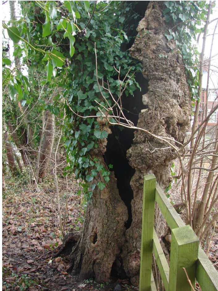
The open split on the northwest side of the trunk at Target Note 2 .
