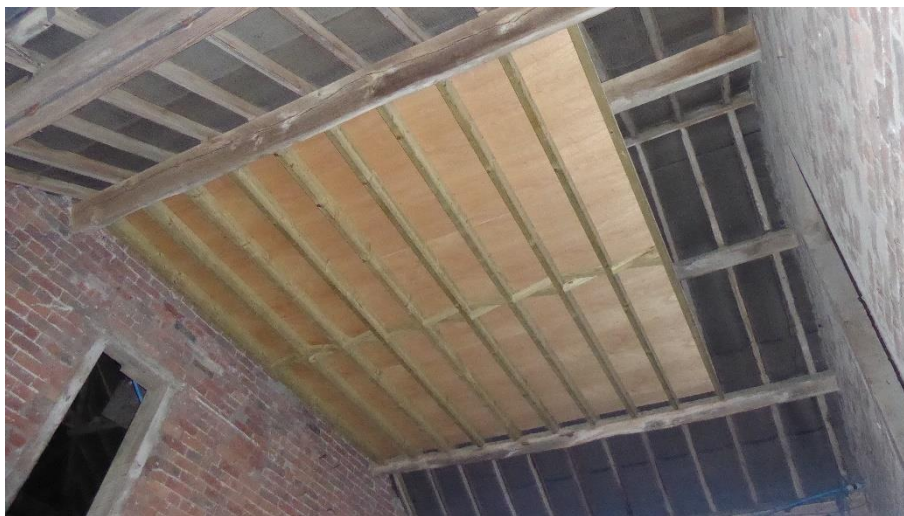
Figure 5.1. The loft floor has already been installed
