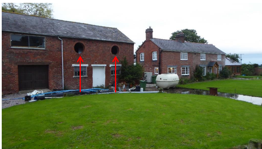
Figure 5.5. Accesses into the loft which will be enhanced with swallow cups
