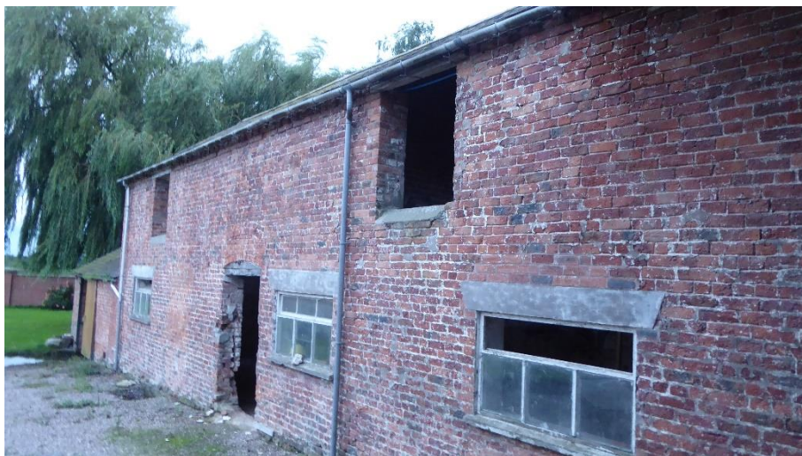
Figure 4.2. Northern side of barn
