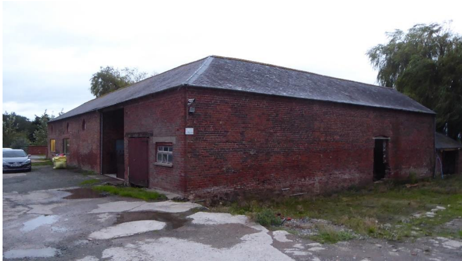
Figure 4.1. Barn from south
