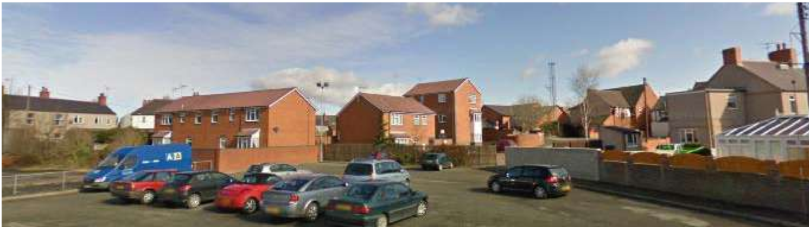
View from the centre of Bonc Wen car park to the north-east.
