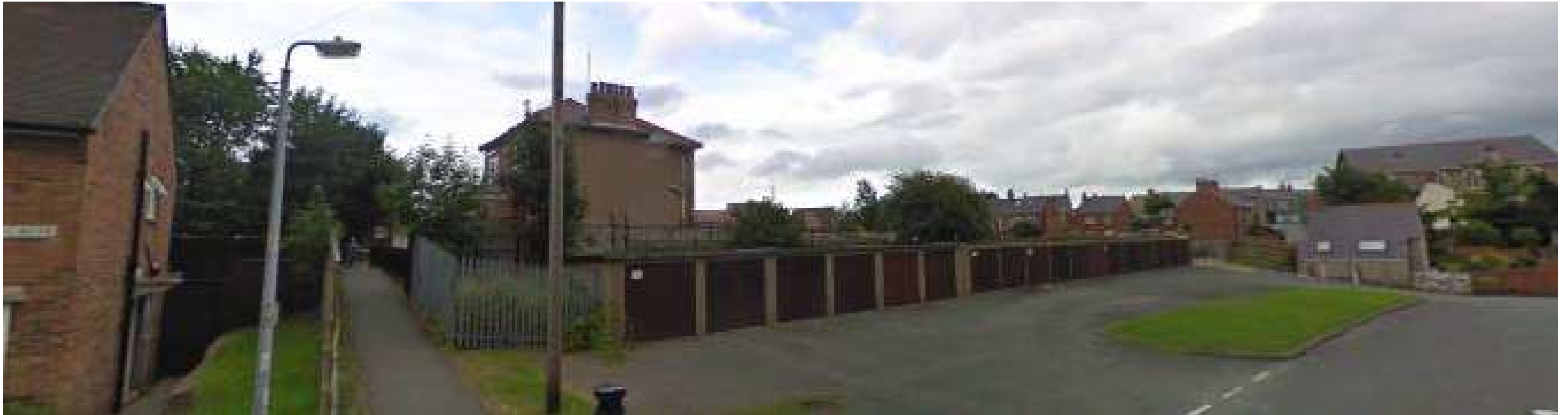
View from Glanrafon towards the site from the west (showing the now demolished building in the centre of the site).
