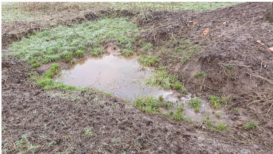
Figure 2.2. Opening of drain
