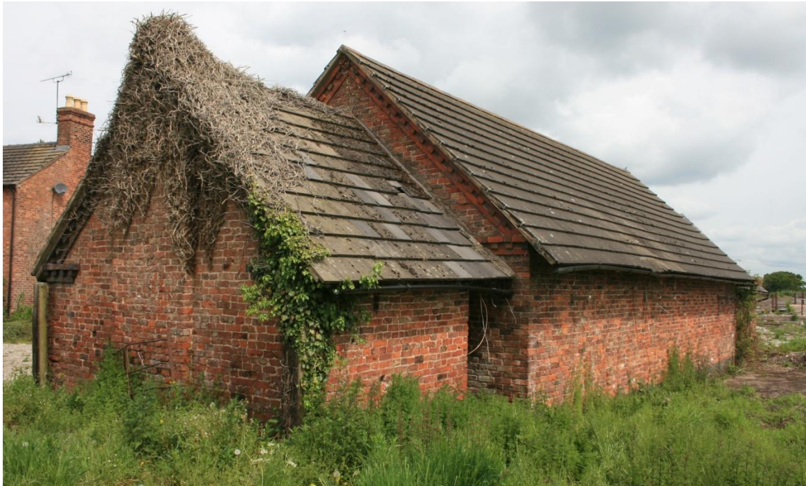
Barn B, south-east corner, showing south extension and its privy entrance, and repetition of the gable detail
