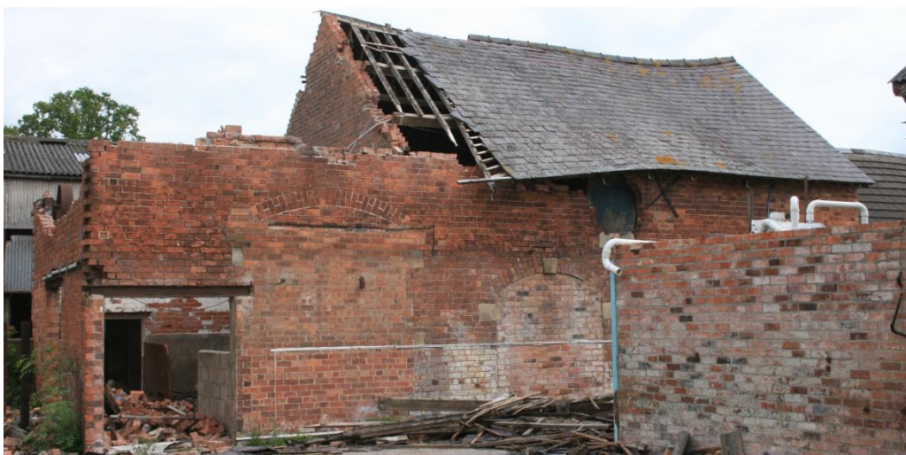
The two-storey western end of the 1879 range: south (yard) elevation showing the extra high doorway for a portable steam engine, an inserted doorway to its left
