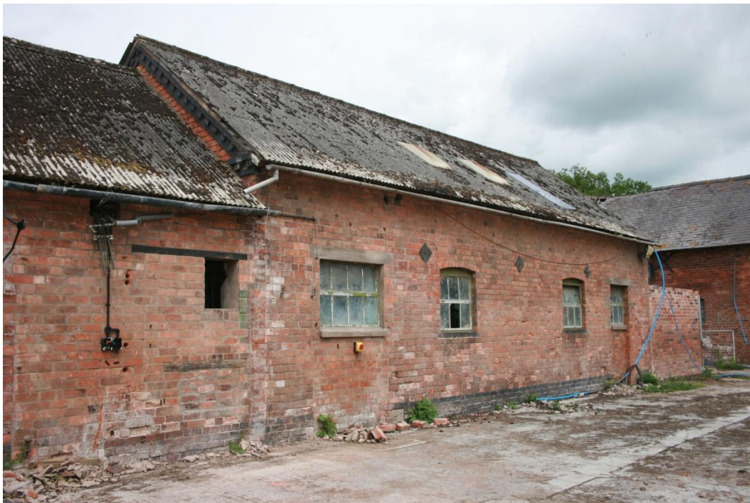
Barn 'A' farmyard (east) elevation showing the main block with extensions added at both ends, that at the south end (nearest the camera) partly covering the engineering-brick gable pediment detail
