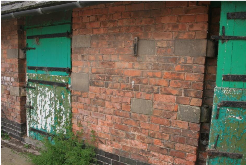
'Barn C', stable block. Detail of yard elevation showing doors, their furniture and supporting masonry blocks
