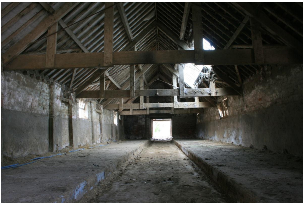
The 'L-shaped barn' 1879 north range. Top: view looking west along the rear (north) wall; bottom: the cow house interior, looking west, some of the original door positions can be seen from their projecting reveals (left)
