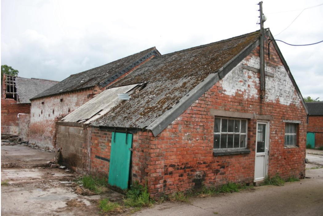
'Barn A' view from south-west corner, dairy in foreground
