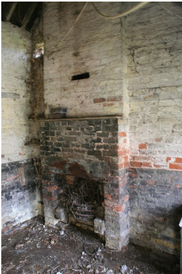
Barn B, interior and fireplace of the heated and glazed room in the south extension
