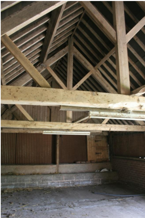
Barn B: left: interior with modern roof, looking south; right: one of the jowled arcade posts
