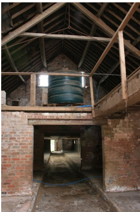
The 'L-shaped barn' 1879 north range. Top: the yard elevation showing signs of five blocked doorways( note interruptions of the base courses); middle: the integral drive shaft in the engine bay passing through the wall into the feed loft; bottom: the partly-unfloored feed loft in the two-storey block, looking east into the cowhouse through an inserted or enlarged doorway
