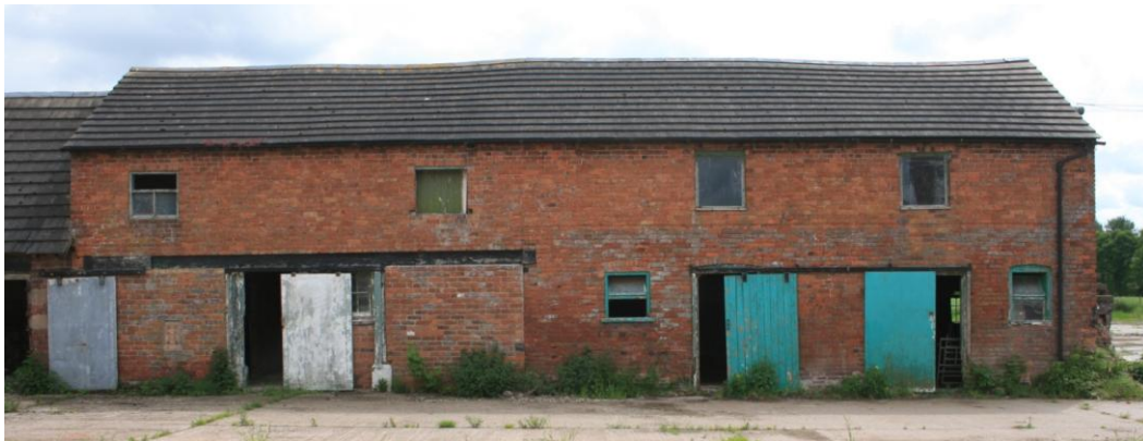
The east range, farmyard (west) elevation. This is the earliest standing building on site. It consists of an open-arcade cart-shed (left) and loose-boxes (right) under rooms for grain or bedding storage
