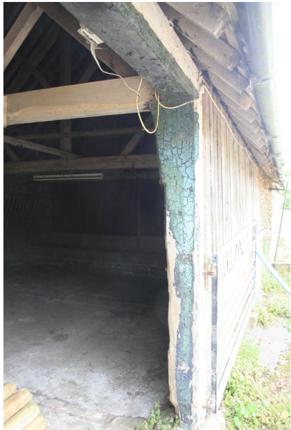
Barn B: left: interior with modern roof, looking south; right: one of the jowled arcade posts
