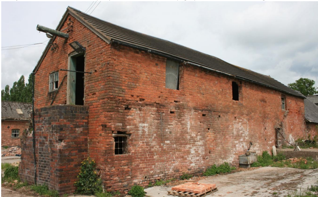
The 'L-shaped barn' east range, rear/east elevation. Note the gable scar of a removed wing that projected from the far (north) end
