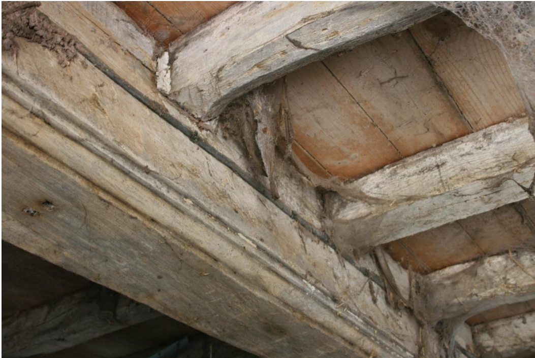
'L-shaped barn', east range, loose-box ceiling showing one of the second-hand moulded cross-beams with the mortices for a previous set of (wider) joists infilled with plaster
