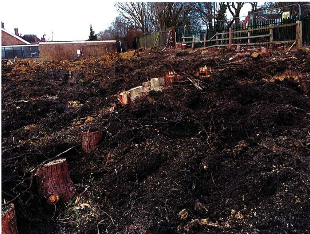
Photograph 3 looking north post demolition
