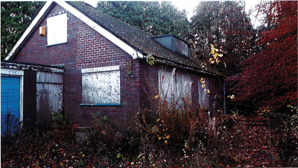
Photograph 1 Previous Bungalow on site
