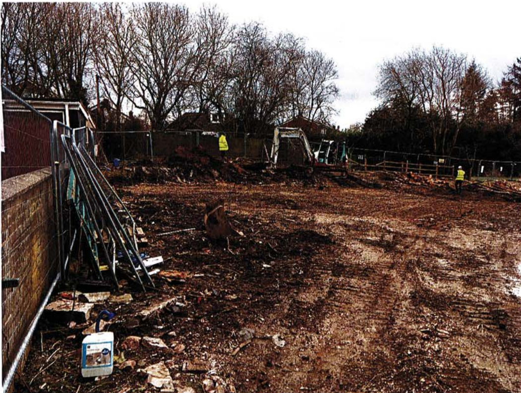
Photograph 12 north east corner of site at plotted shaft location
