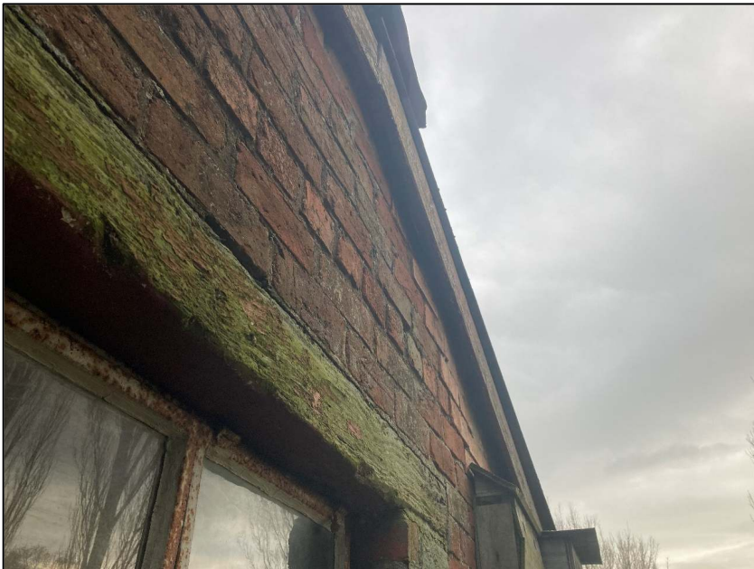
A1.8 Plate 8: Bargeboard on eastern gable aspect
