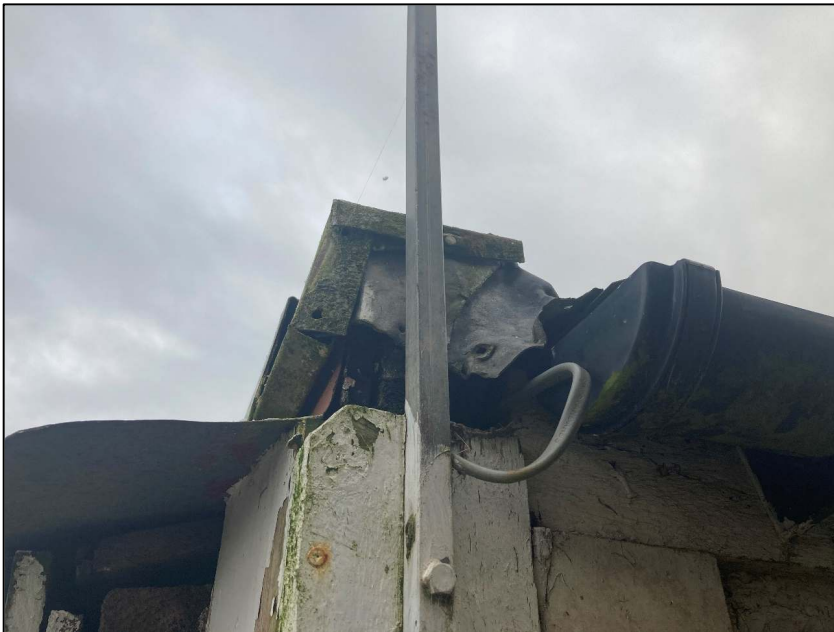
A1.6 Plate 6: Example of gap between fascia board
