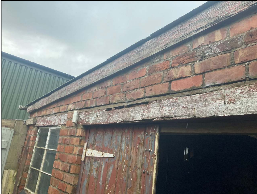
A1.8 Plate 8: Bargeboard on eastern gable aspect
