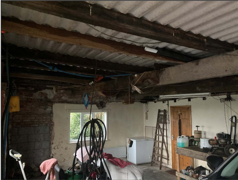
A1.11 Plate 11: Interior of section 2 of building
