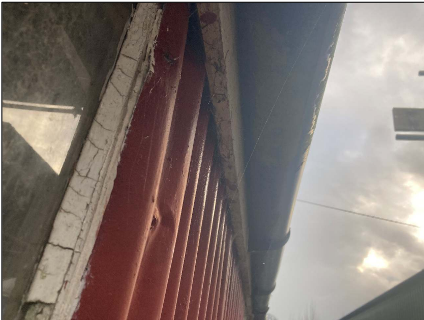
A1.4 Plate 4: Example of gaps behind fascia boards on southern aspect of building
