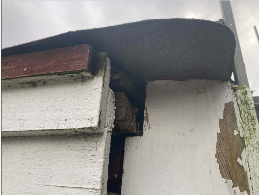
A1.6 Plate 6: Example of gap between fascia board
