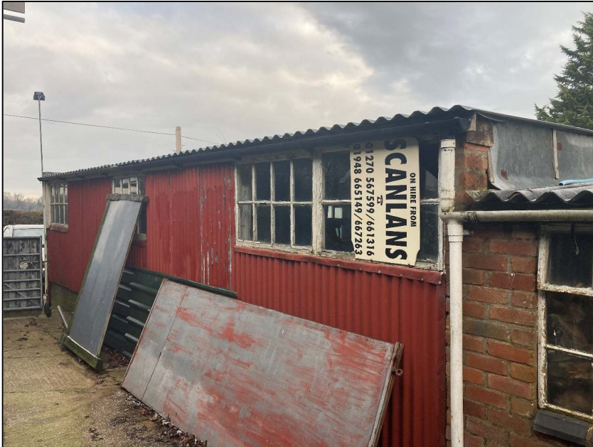
A1.4 Plate 4: Example of gaps behind fascia boards on southern aspect of building
