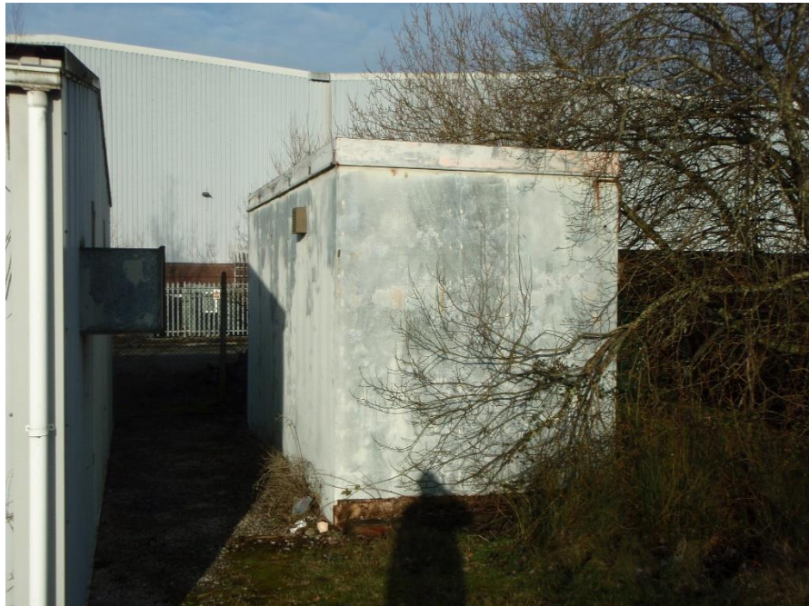
Structure at Target Note 1d .
