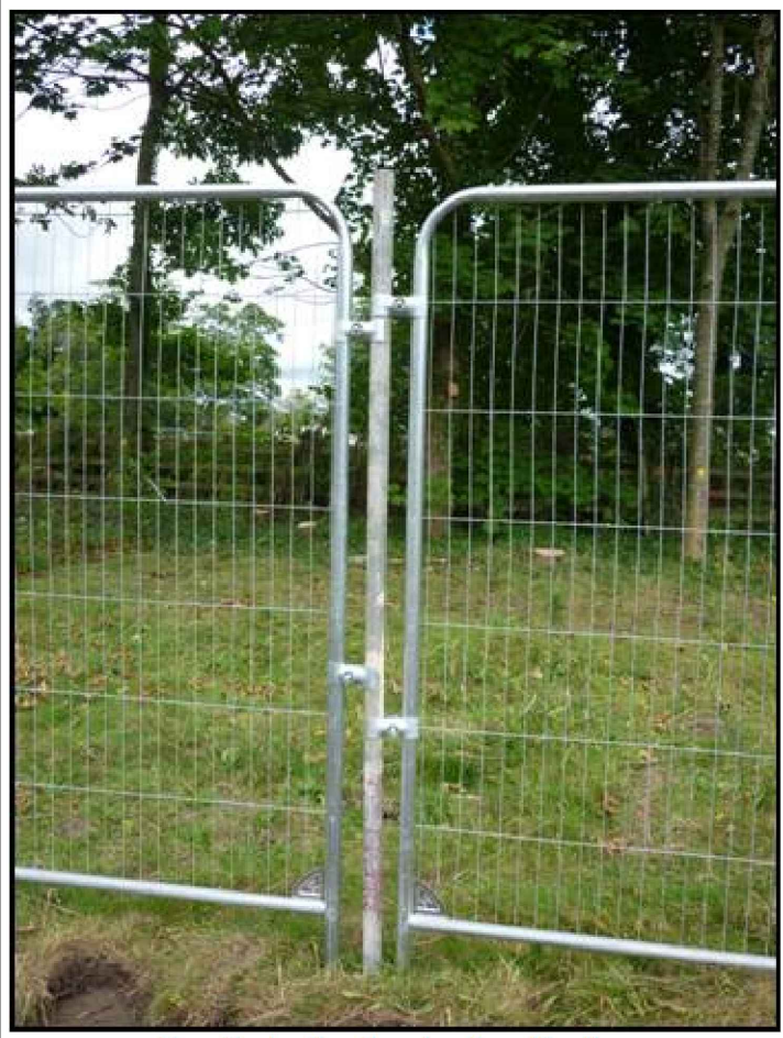
Tree Protective Fencing Specification
