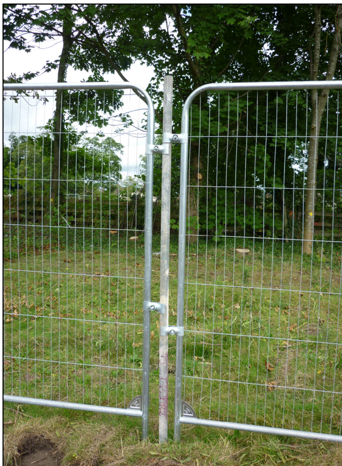
Tree Protective Fencing Specification
