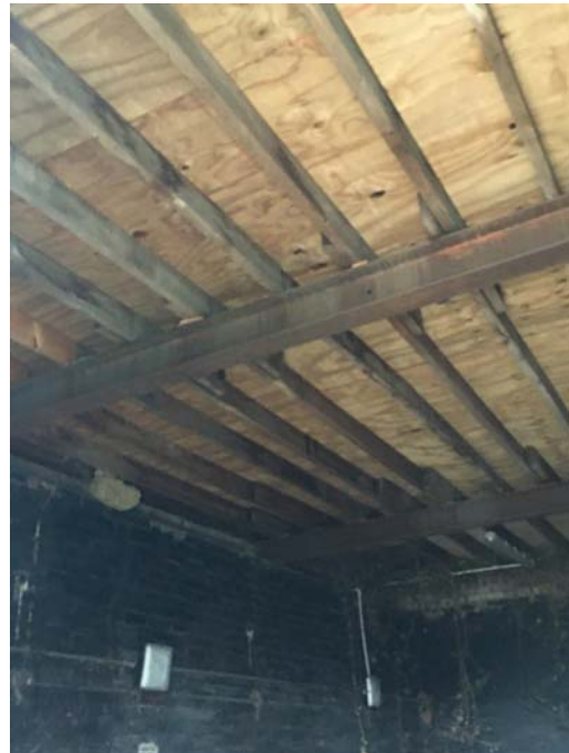
Photograph 12 – Interior of Building P2-B2 showing exposed roof structure.
