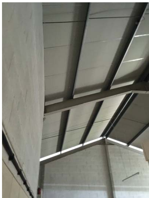
Photograph 5 – Interior of Building P1-B1 showing exposed roof structure
