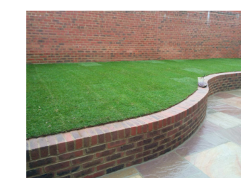
3 - Low Level Br Retaining Wall
