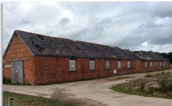
Above: Main Outbuilding
