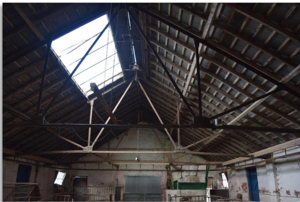
Above: Inside Main Outbuilding
