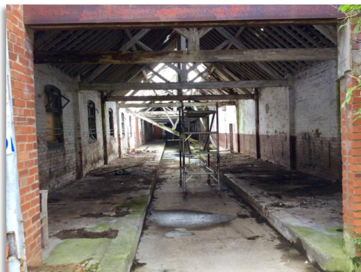
Above: Inside Main Outbuilding
