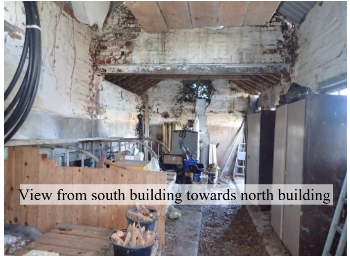
View towards south building
