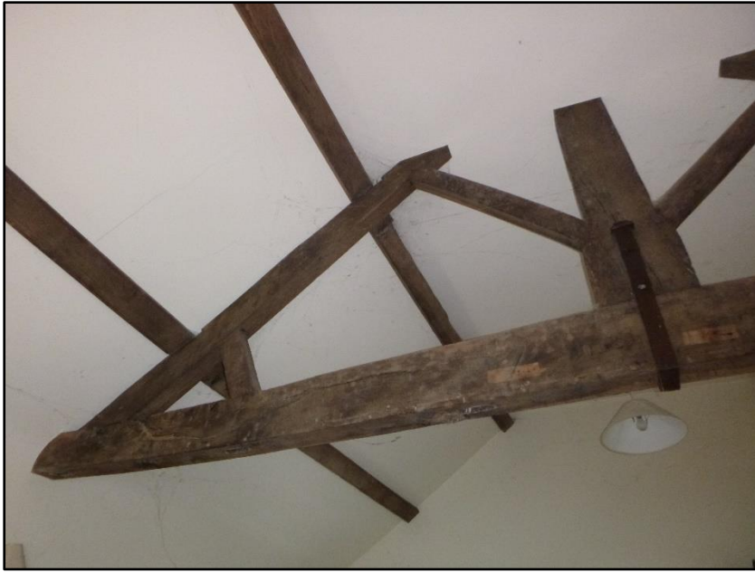
Photograph 4 showing first floor room
