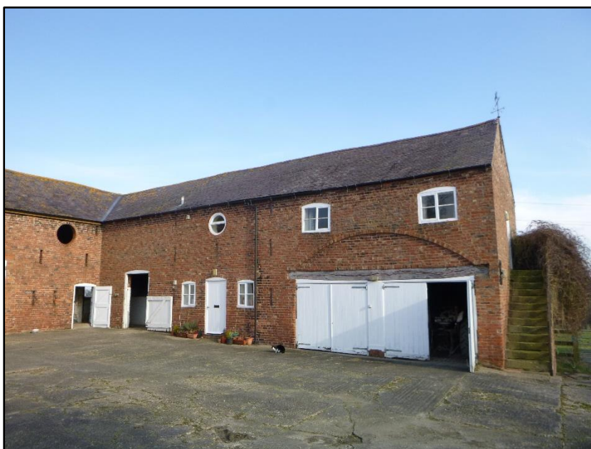
Photograph 1 showing the exterior of the barn
