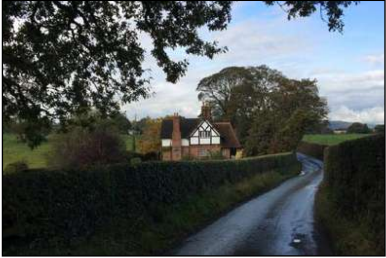
Context photo of 1 residential property called the Elms Cottage off Vicarage Lane
