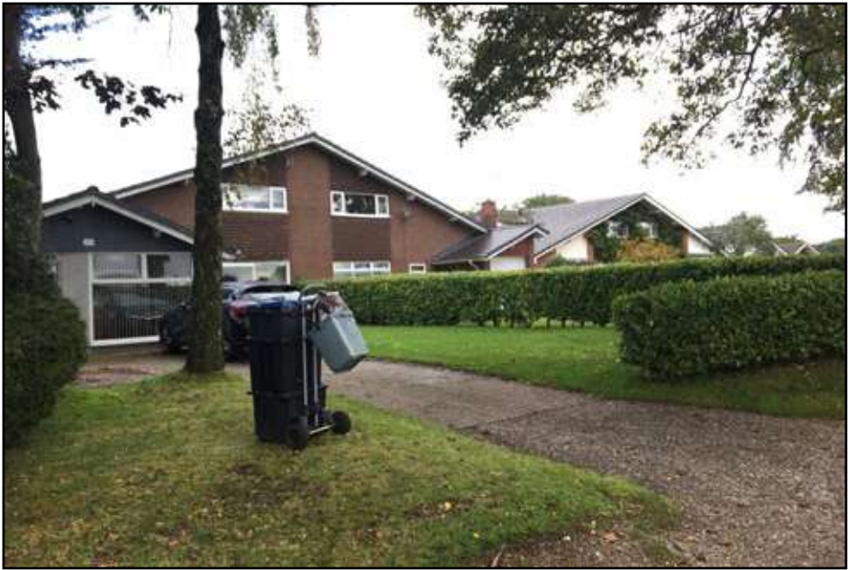
Context photo of residential properties off Hillock Lane set back by large gardens and drives.
