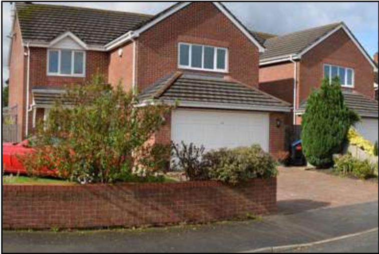
Context photo of 2 residential properties at end of Stancliffe Avenue facing east.
