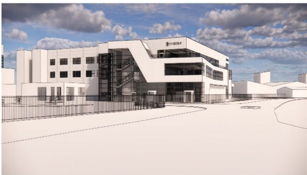
Figure 8 - View toward Building One, as existing
