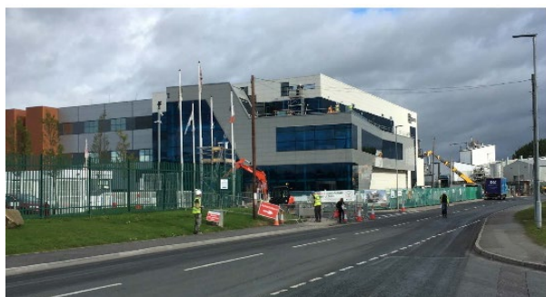
Figure 9 - Comparison photo towards Building One, as existing
