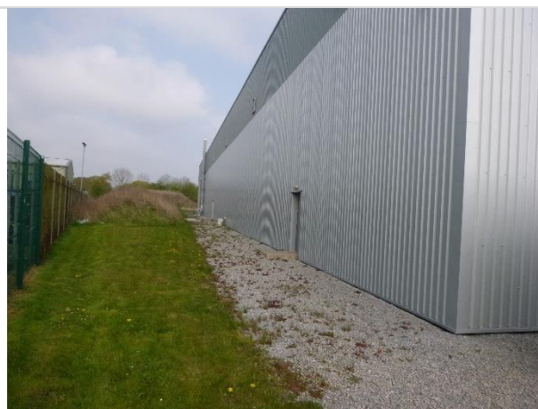
Photo 6: Amenity grassland south of Building 1 (facing west)
