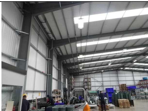
Photo 13: Interior of Building 2 showing western aspect (facing north-east)
