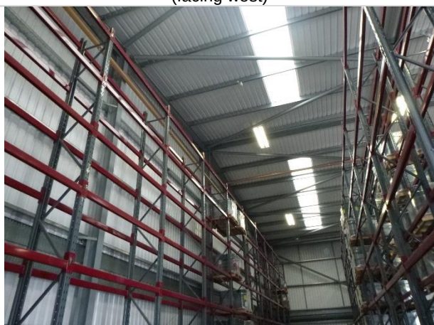
Photo 11: Interior of Building 1 showing southern aspect (facing west)
