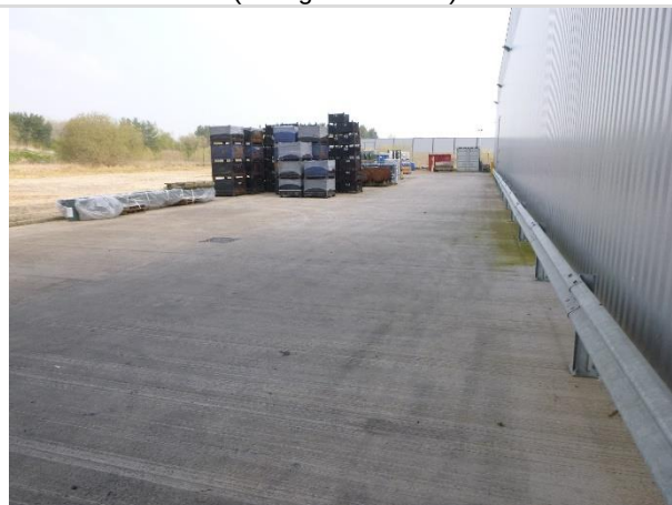
Photo 4: Hard standing (facing north-east)
