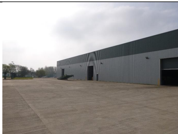
Photo 8: Hard standing and northern aspect of Building 1 (facing south-east)
