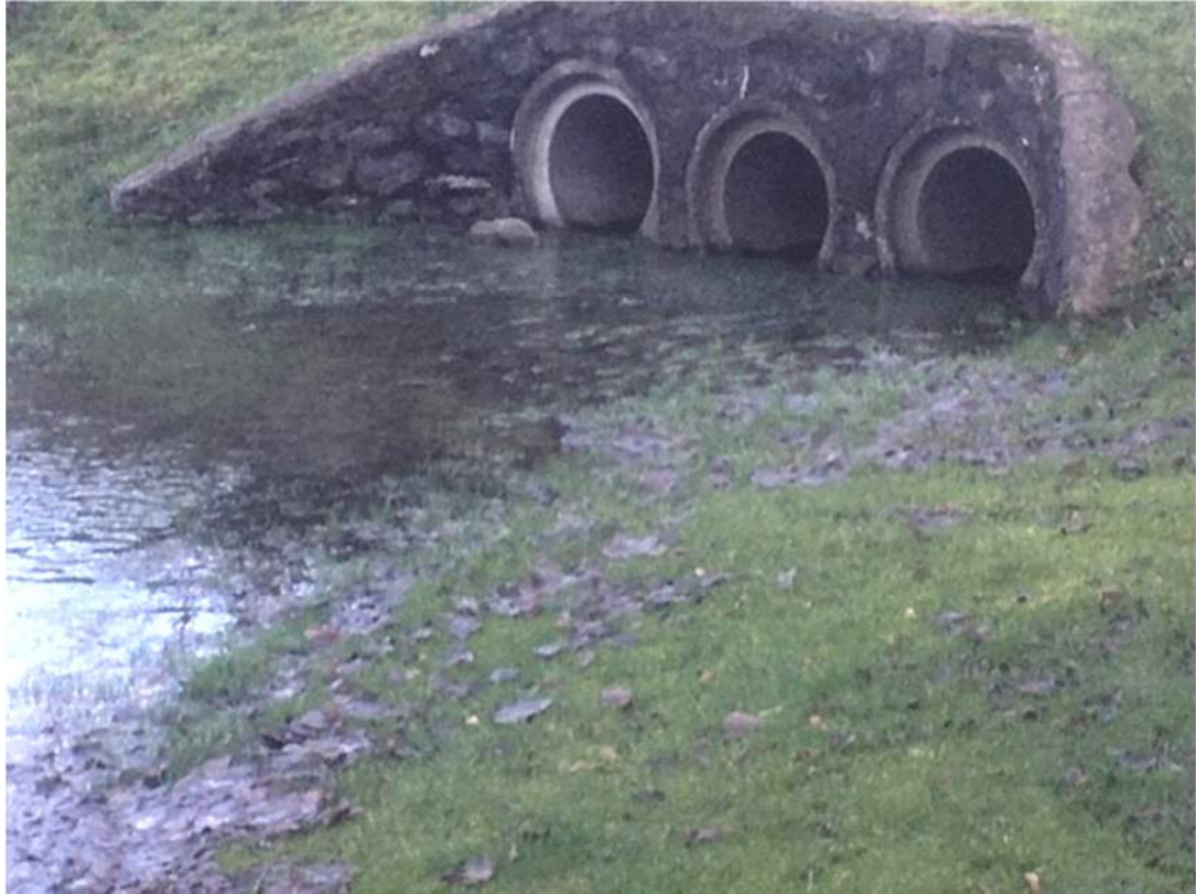
PHOTOGRAPH 1 3 x 825mm pipes passing from the Site under the B4500
