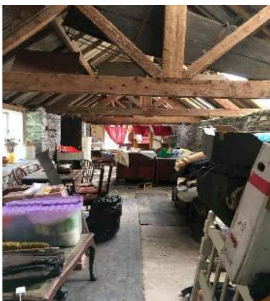
PR10: View of internal structure showing king post beams
