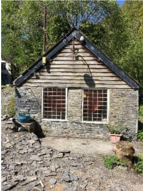
PR1: East gable showing weather boarding and fascia
