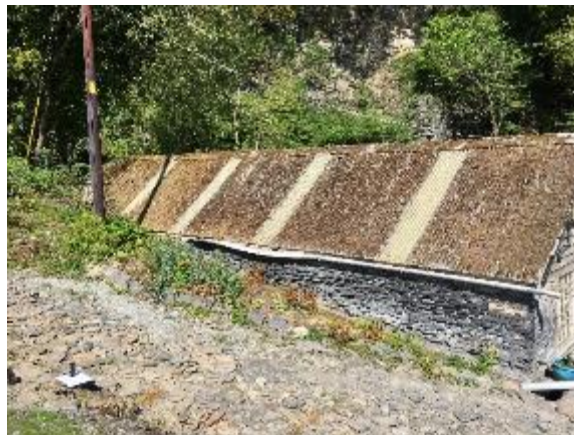
PR4: South elevation and asbestos roof
