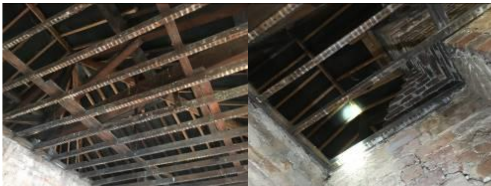
Plate 5: Internal character of the second floor with exposed loft
