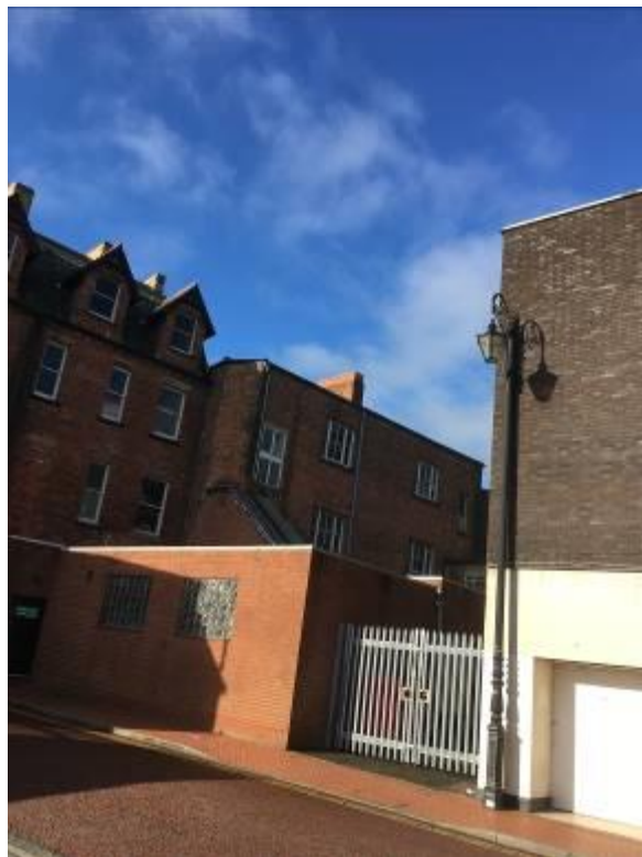
Plate 2: Rear elevation of the building
