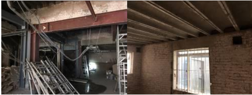
Plate 3: Internal character of the ground floor
