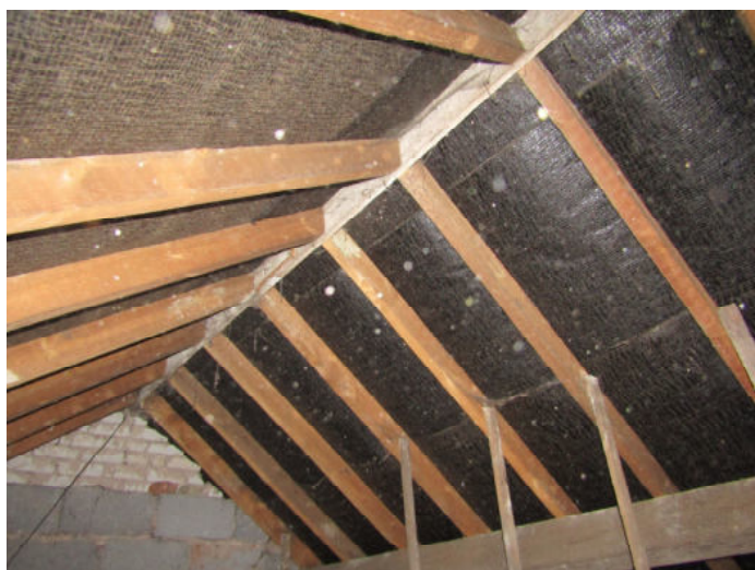
Photo 2: 1F Bitumastic felt beneath slates and cobwebs covering roof timbers.
