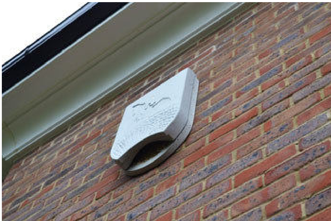
Figure 6: Schwegler (1FQ) bat box fitted to wall.
