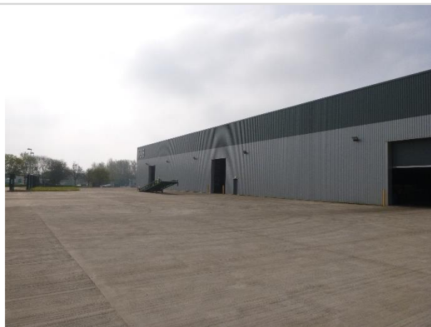
Photo 8: Hard standing and northern aspect of Building 1 (facing south-east)
