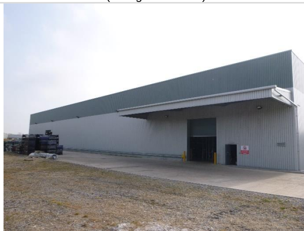
Photo 12: Hard standing, colonising vegetation and western aspect of Building 2 (facing east)
