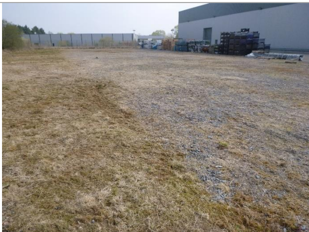
Photo 1: Vegetation colonising compacted hard standing (facing north-east)
