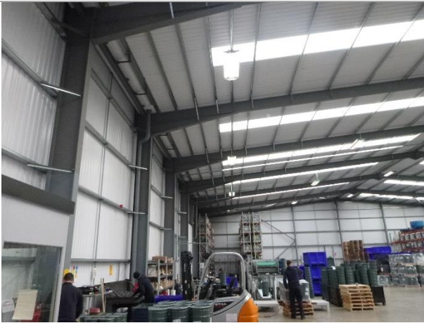
Photo 13: Interior of Building 2 showing western aspect (facing north-east)
