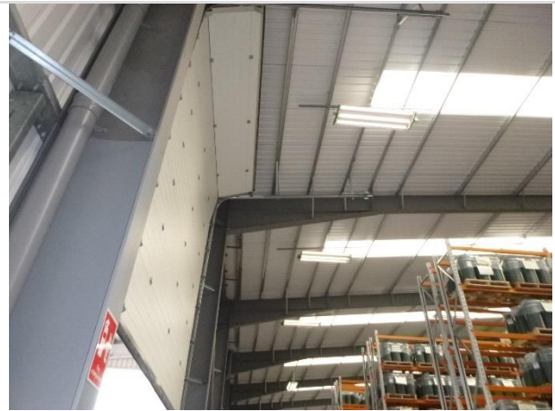
Photo 14: Interior of Building 2 showing western aspect (facing north-east)
