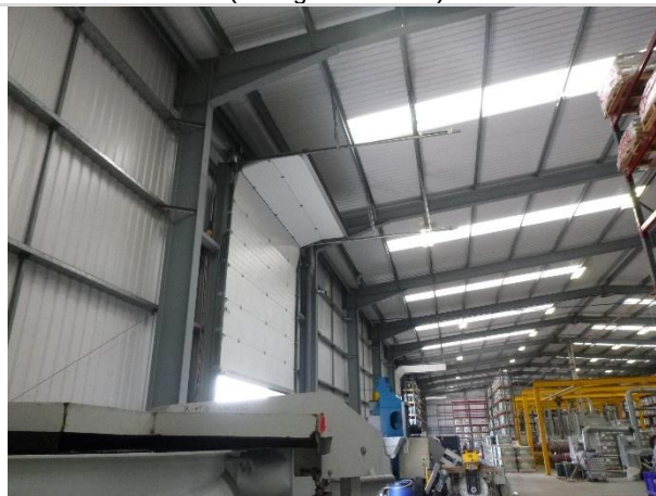
Photo 10: Interior of Building 1 showing northern aspect (facing south-east)
