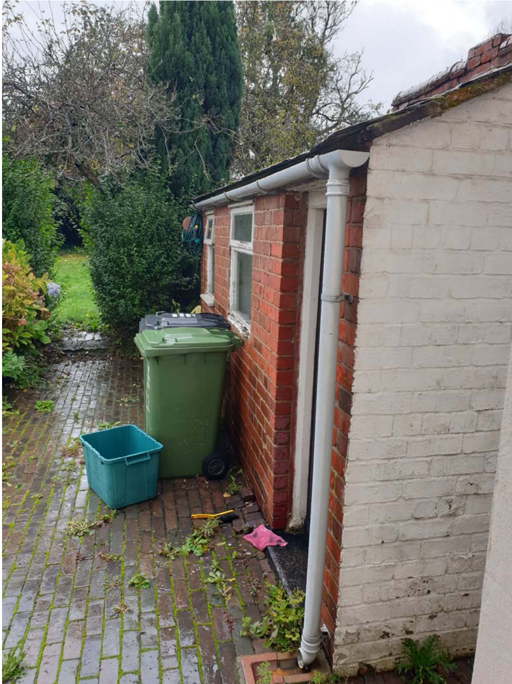
Photos of the Existing Outbuilding & Garage
