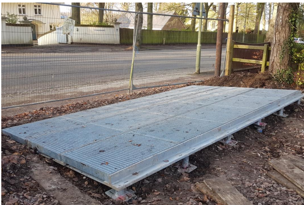
Figure 5. An example of a proprietary root bridge product under construction.
