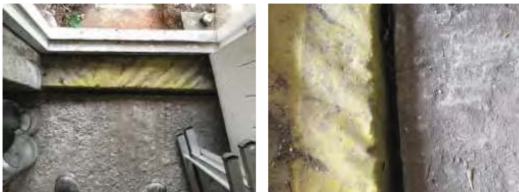
Figure 4 - Slab movement
