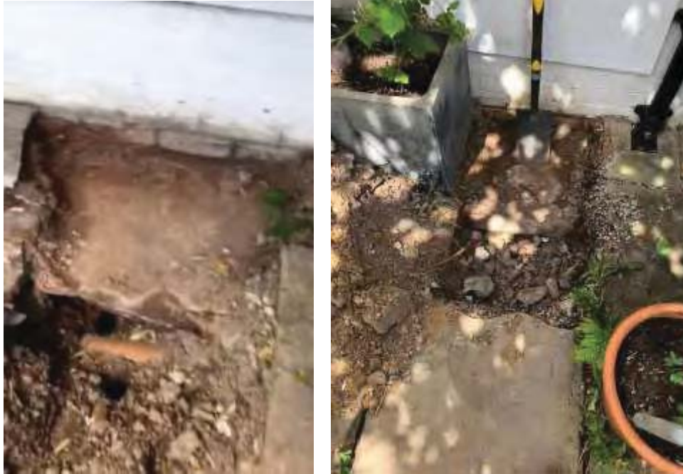
Figure 5 - Exposed Concrete Foundations
