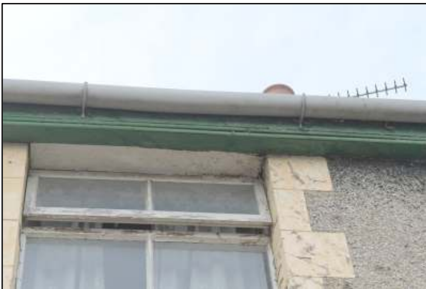
Sealed timber soffits at the front
