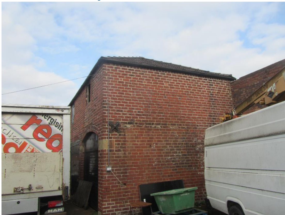
Image 3.25 Western elevation of B3
