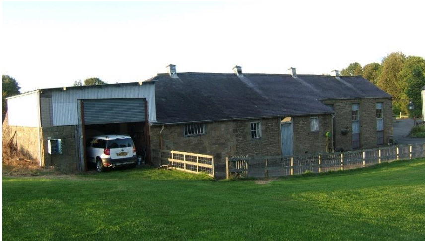
Figure 5.10 Photograph of Outbuilding 3 – North Elevation
