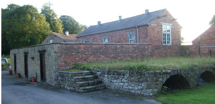
Figure 5.6 Photograph of Outbuilding 2 – North Elevation
