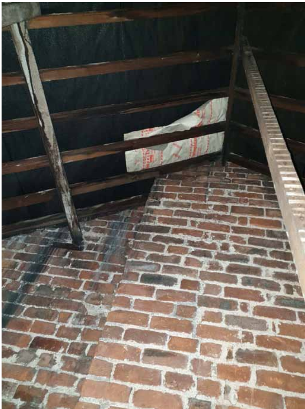
Photographs of Existing Roof void & Roof light Insertion Locations
