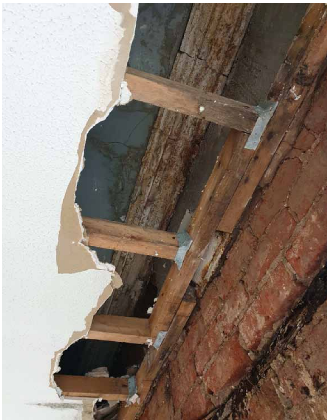
Photographs of Second Floor Suspended Ceiling & Roof Void To Frontage
