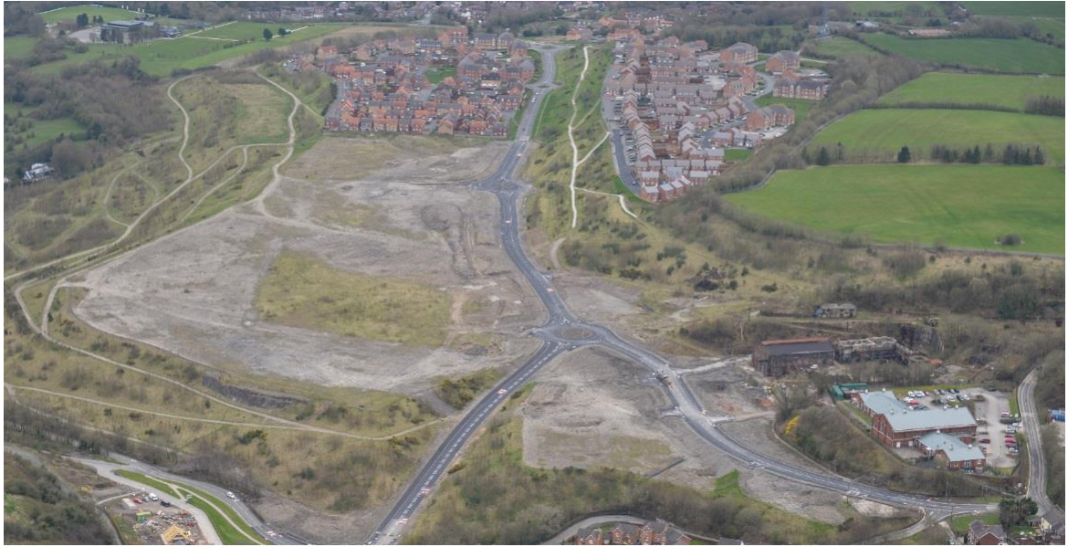
Figure 1: Image of the existing site – looking south
