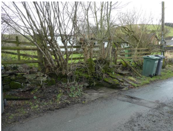
Photo 6: north boundary (laneside) of NE corner
