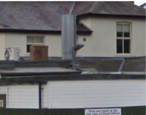
Previous Existing Stainless Steel Flue Approx Height 1500m above roof line
