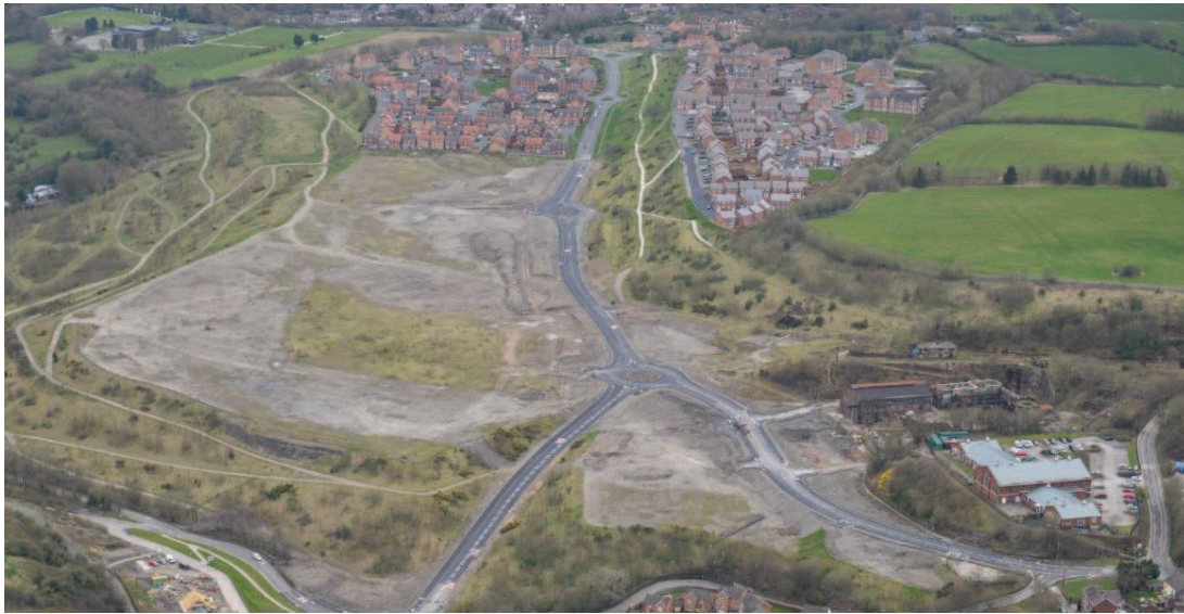
Figure 1: Image of the existing site – looking south
