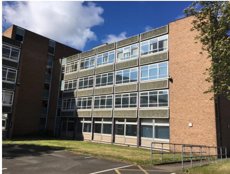
Plate 1: North-West elevation of the Crown Buildings
