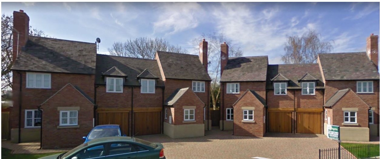
Fig.6 Recently completed new housing.
