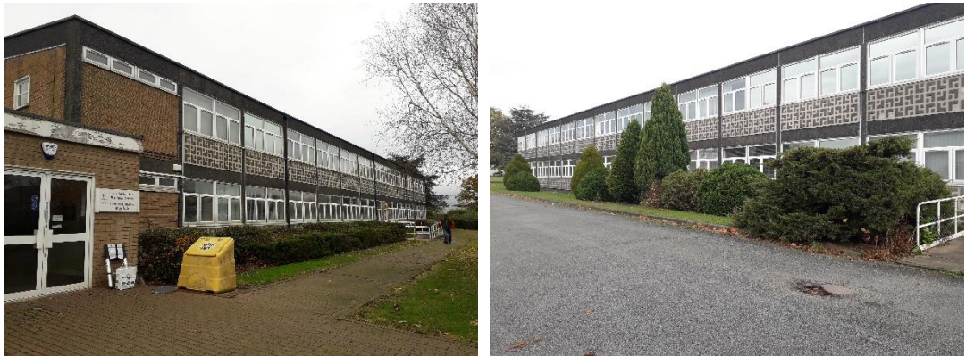
Photos 4.1 & 4.2: The eastern and western elevations of the two-storey section ( Target Note 14 in Marches Ecology, 2020 )
