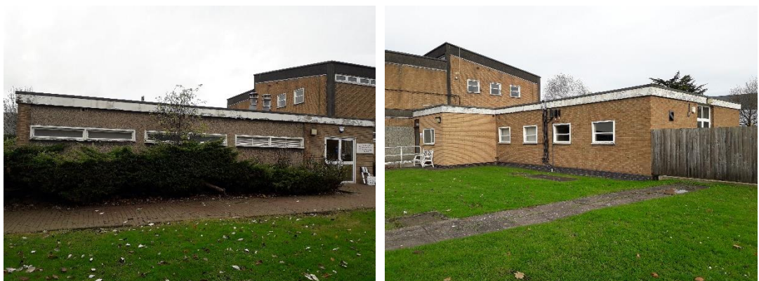
Photos 4.3 & 4.4: The eastern and western elevations of the single storey section ( Target Note 14a in Marches Ecology, 2020 )
