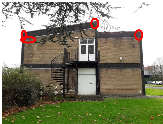
Photo 4.7: Location of potential roosting features on the northern elevation of the building
