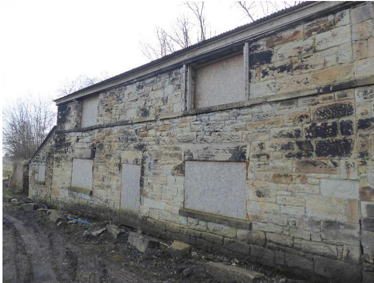
PHOTO 4.1 NORTHERN SIDE OF THE HOUSE
