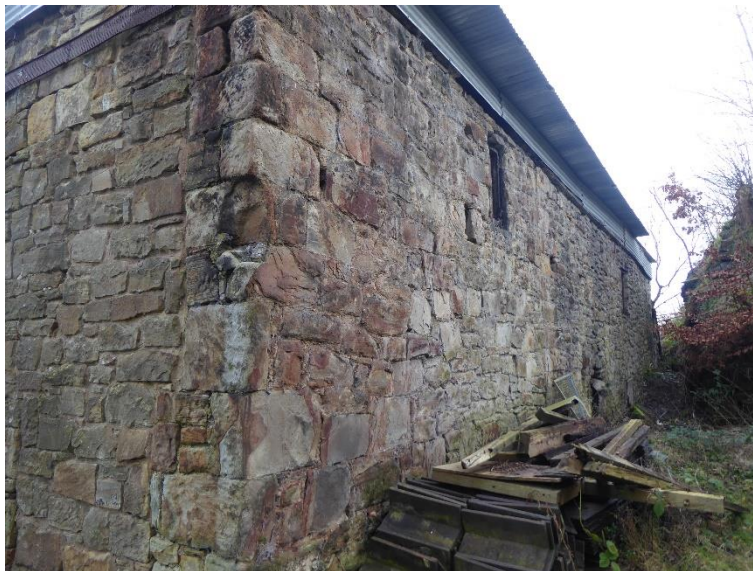
PHOTO 4.2 SOUTHERN SIDE OF THE HOUSE
