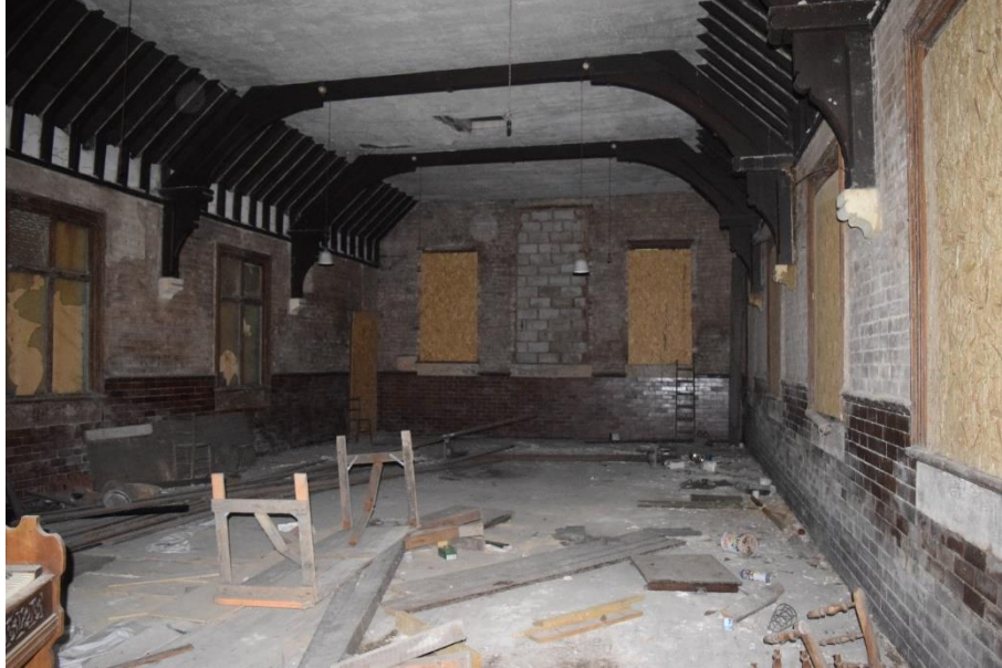
Figure 4.5. Interior of school room
