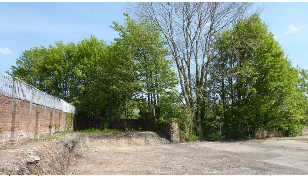
Photo looking towards north of site
