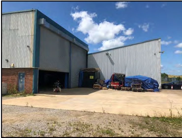
Photograph 3: Main building on site, B1
