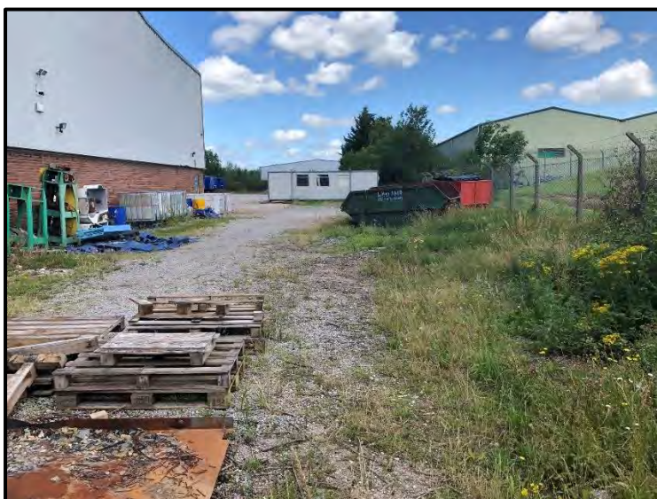
Photograph 2: Portacabin outbuilding, B2
