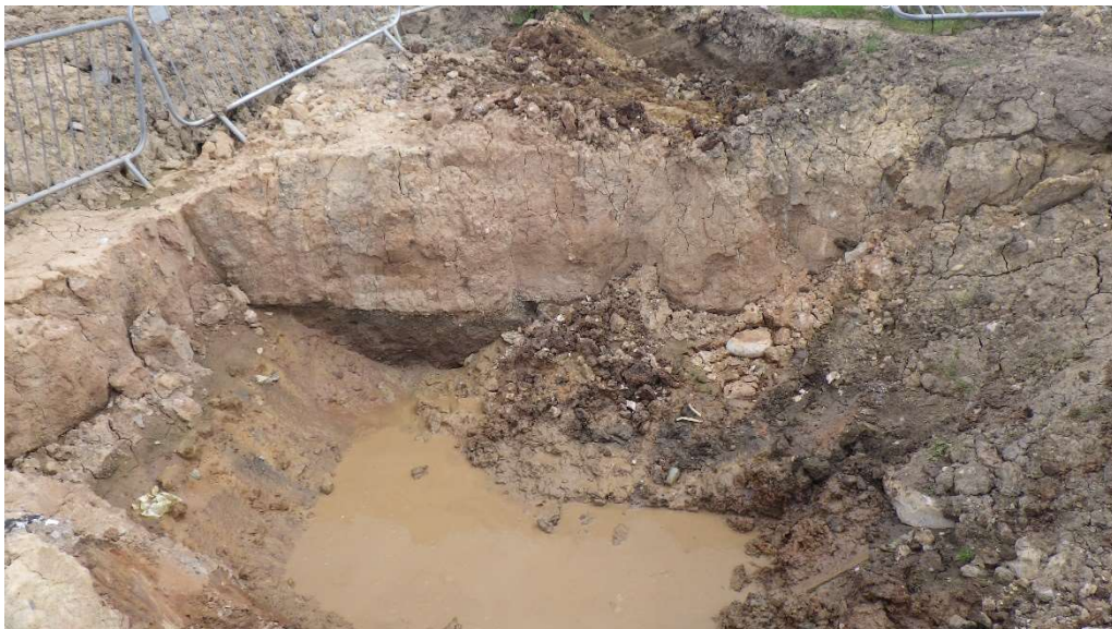
Photo 6 – Completion of the excavation
