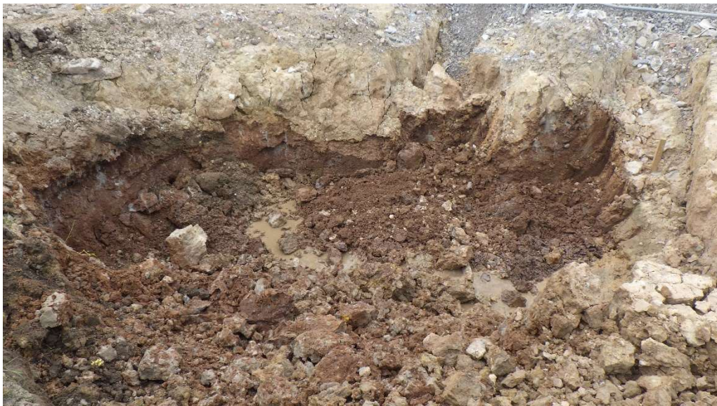
Photo 8 – Further backfilling works
