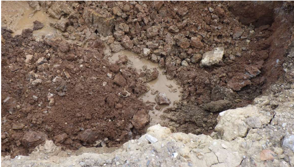
Photo 7 – Backfill of the excavation using natural clay arisings generated from the groundworks
