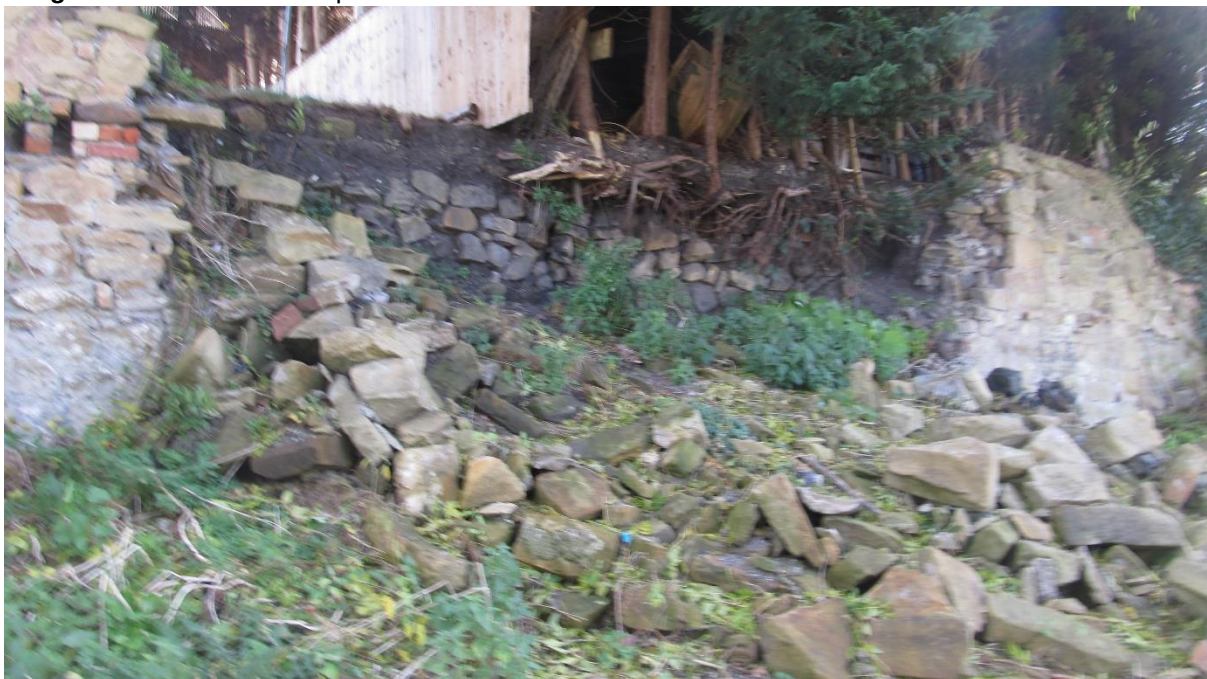
Image 3.9 internal wall collapse
