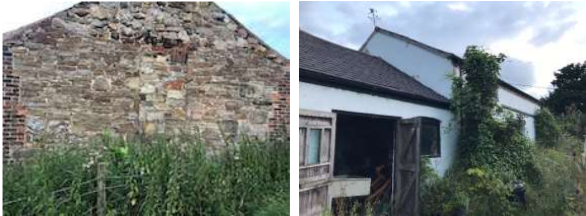
PHOTO 4.3 & 4.4 WESTERN AND EASTERN GABLE ENDS
