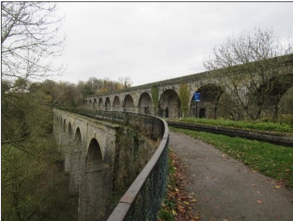
Plate 8: View of Chirk Aqueduct and Canal
