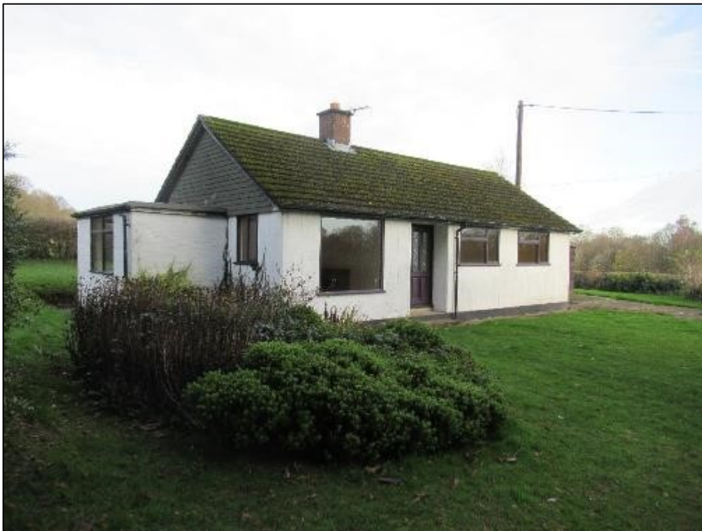
Plate 1: View across the Site towards the north east
