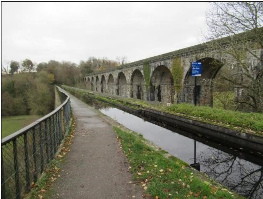
Plate 6: View of Chirk Aqueduct and Canal
