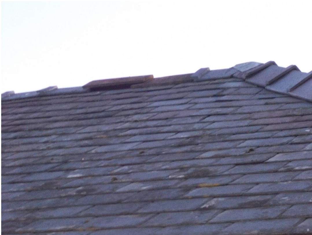
Plate 4: A photograph of an air ridge on the roof of barn 'B1'.
