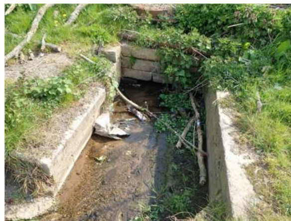
B5425 Culvert Inlet ESTRY Unit: Circular Culvert
