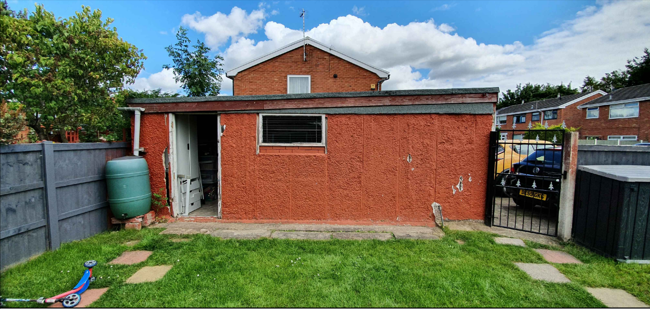
07. Photo of existing garage
