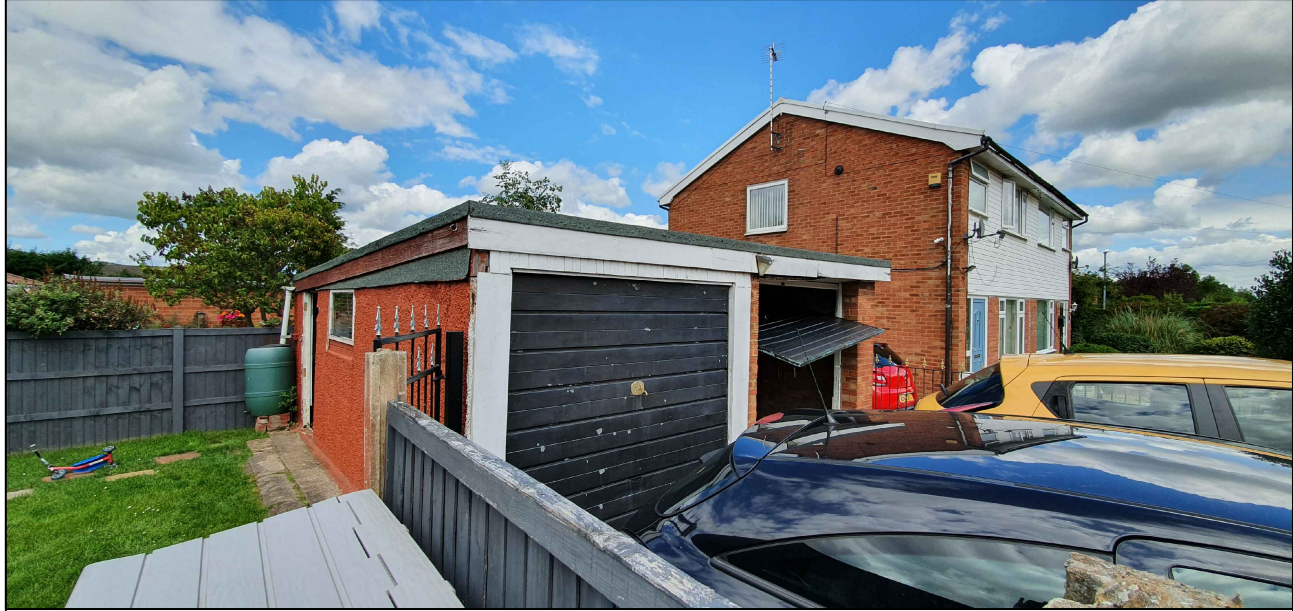
06. Photo of existing garage
