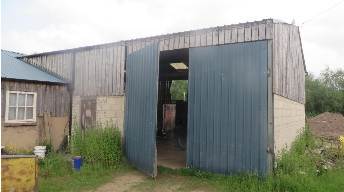
Image 3.5 The eastern portion of B1 with timber cladding, corrugated metal roof and breezeblock base
