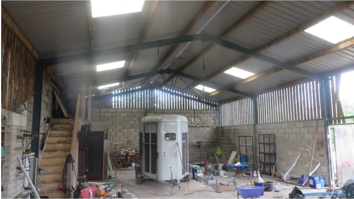
Image 3.9 Eastern portion of B1 with steel roof supports and light infiltration, unsuitable for bats
